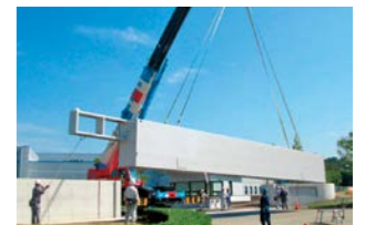
Building a circumferential seawall around the Matsushige Factory
