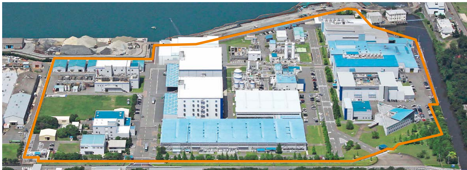
Circumferential seawall ● Total length: 1,620 m ● Height: 2.0 m (T.P. + 3.9 m) on east, west, and south sides; 2.70–3.35 m on north side ● Installation date: June 2014 ● Steel pipe pile: 300–400 mm (diameter); 17–20 m (length); 678 used in total
