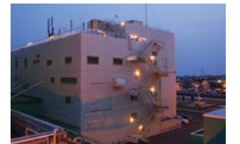
In the event of a power outage, emergency LED lights will automatically light evacuation routes and evacuation centers for more than 20 hours
