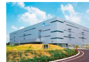
The West Japan Logistics Center, a new BCP-compliant delivery facility, opened in Kobe in 2015 by Otsuka Warehouse Co., Ltd.
