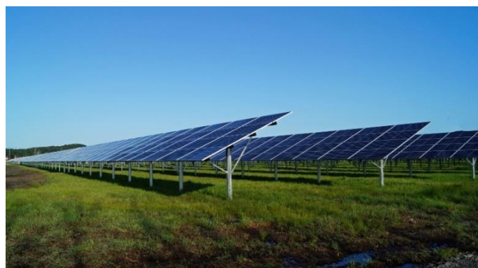
Some of the solar panels installed
