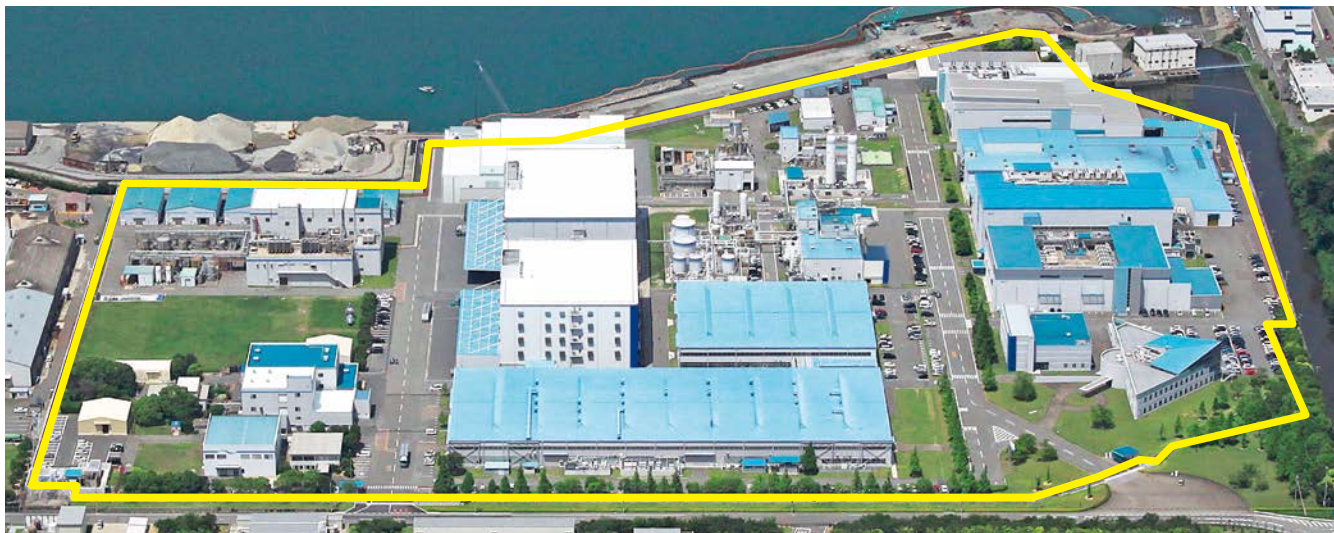
Circumferential seawall ● Total length: 1,620 m ● Height: 2.0 m (T.P. + 3.9 m) on east, west, and south sides; 2.70–3.35 m on north side ● Installation date: June 2014 ● Steel pipe pile: 300–400 mm (diameter); 17–20 m (length); 678 used in total
