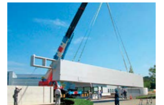
Building a circumferential seawall around the Matsushige Factory
