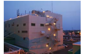
In the event of a power outage, emergency LED lights will automatically light evacuation routes and evacuation centers for more than 20 hours
